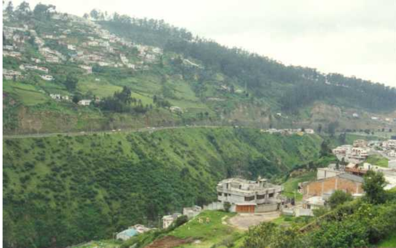
Figure 32. Self-built structures on steep slopes.
