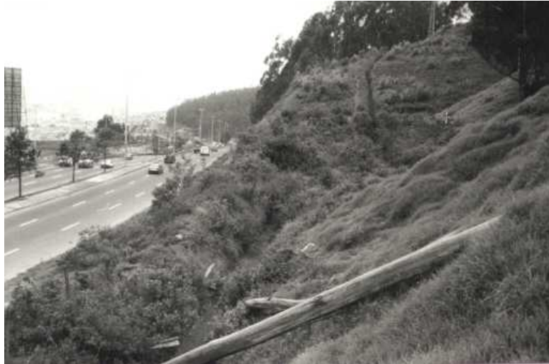
Figure 33. Slopes susceptible to landslides along Vía Oriental.
